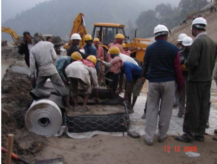
FIG.5: GSCM LINING – PLACEMENT OF GEOTEXTILE FILTER AND G.I. CRATES
