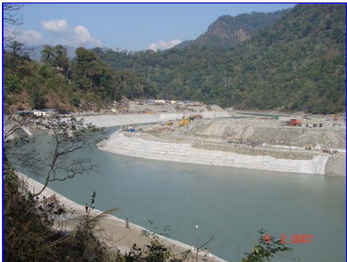
FIG. 1: TEESTA DIVERSION CHANNEL IN GSCM LINING
