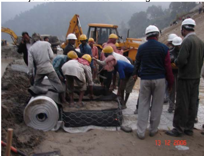
FIG.5: GSCM LINING – PLACEMENT OF GEOTEXTILE FILTER AND G.I. CRATES
