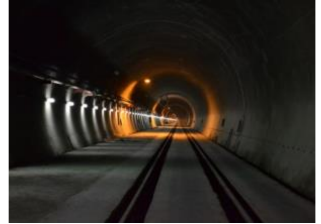
Pir Panjal Rail Tunnel, J&K
