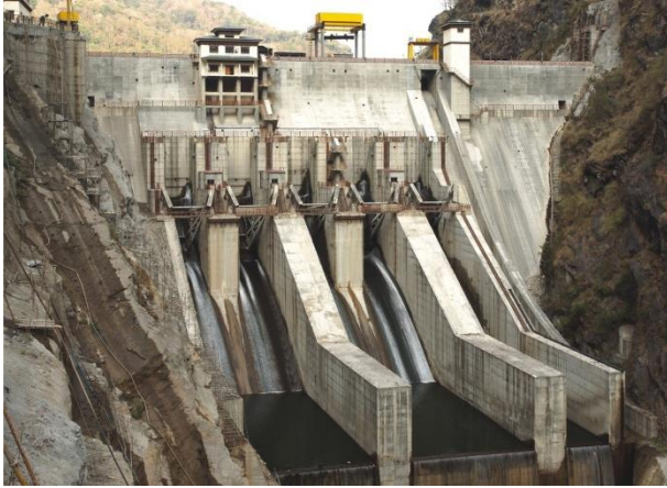
Tala Hydel Power Project, Bhutan
